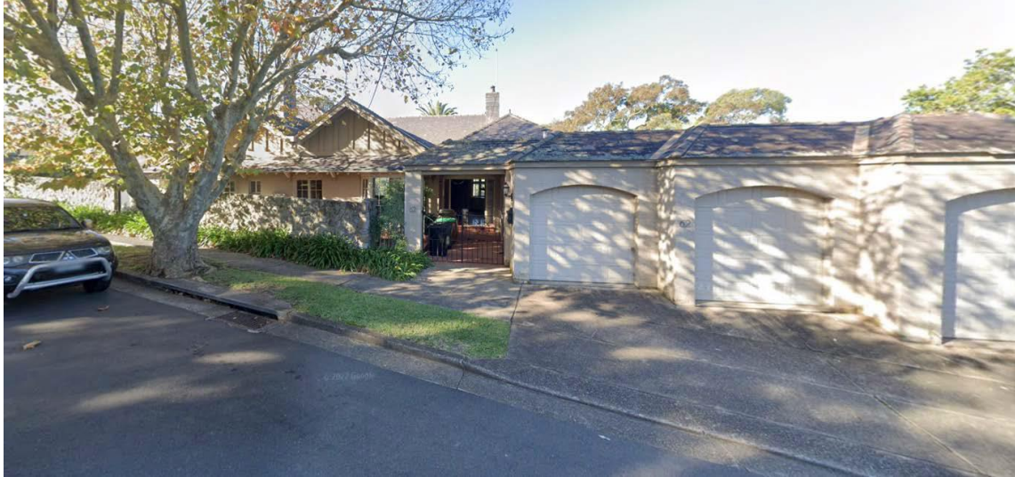
Figure 2 – Dwelling from the Cliff Road frontage, pre-fire.
