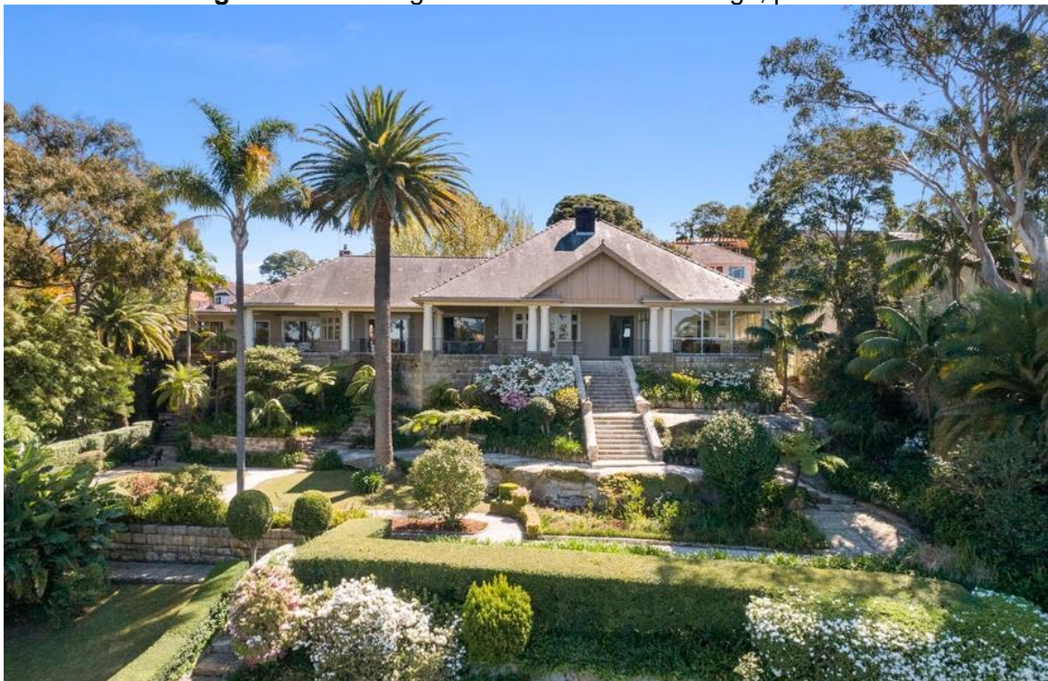
Figure 3 – Dwelling and rear yard, pre-fire.
