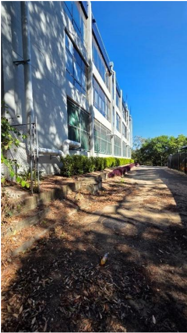
Figure 10. Existing service laneway.
