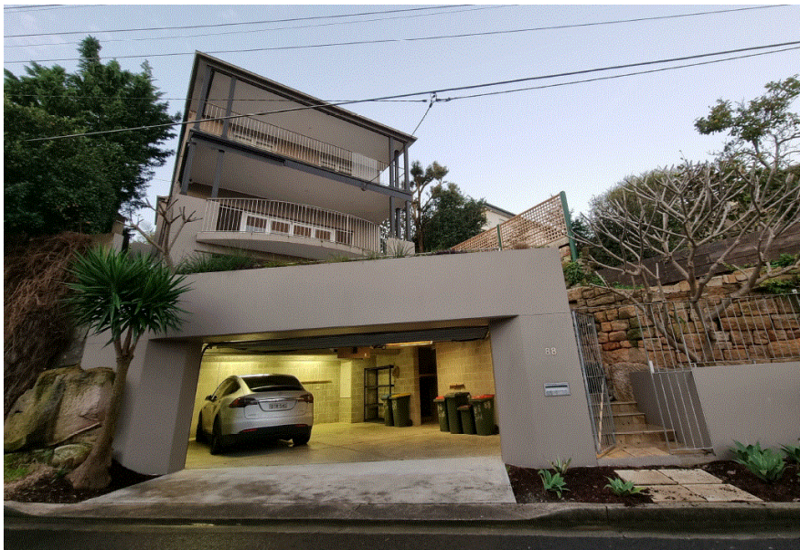
Figure 1: Frontage view from Carlotta Street (Source: Architectural plans)
