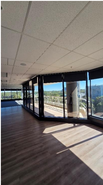
Figure 12. Existing vacant floor and balcony to be converted (level 7).
