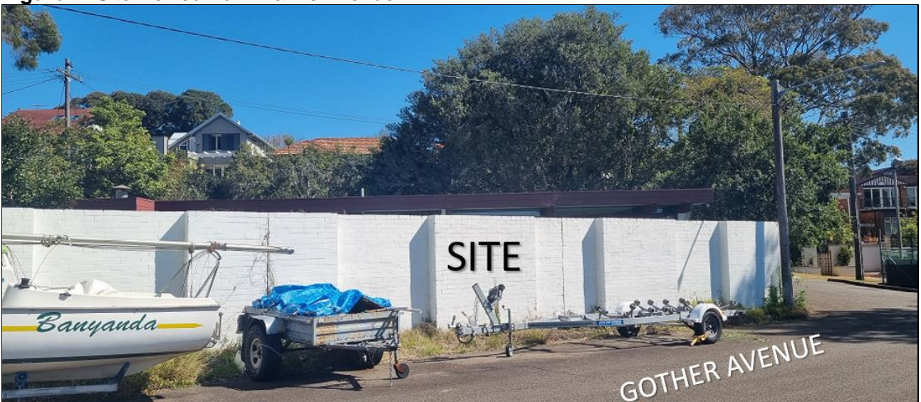
Figure 5: Site viewed from Gother Avenue.
