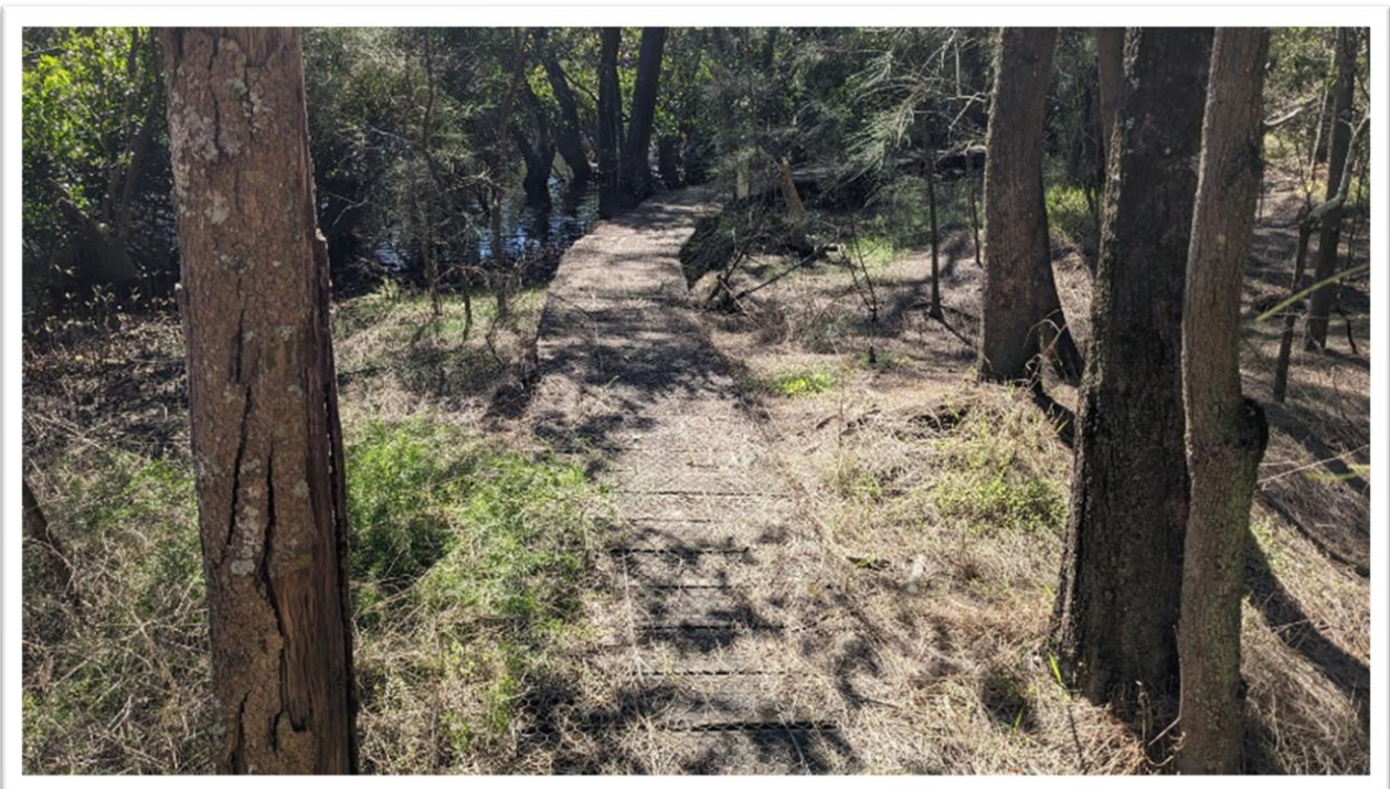
Figure 4: Central Section of Existing Boardwalk Source: DFP EIS
