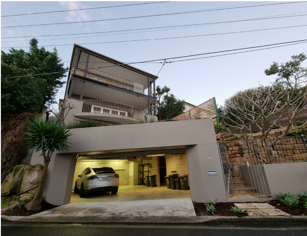
Figure 1: Frontage view from Carlotta Street (Source: Architectural plans)
