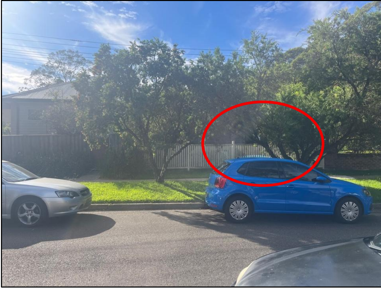
Photo 3: Existing western elevation / location of new carport outlined in red
