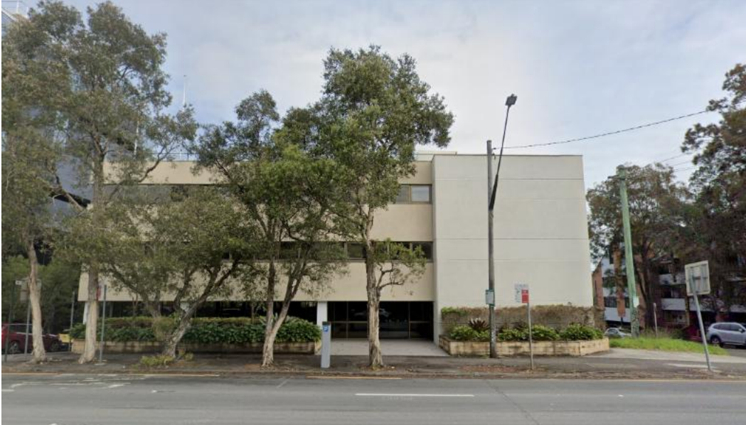
Figure 2: Existing building at 126 Pacific Highway (Source: Google Maps)
