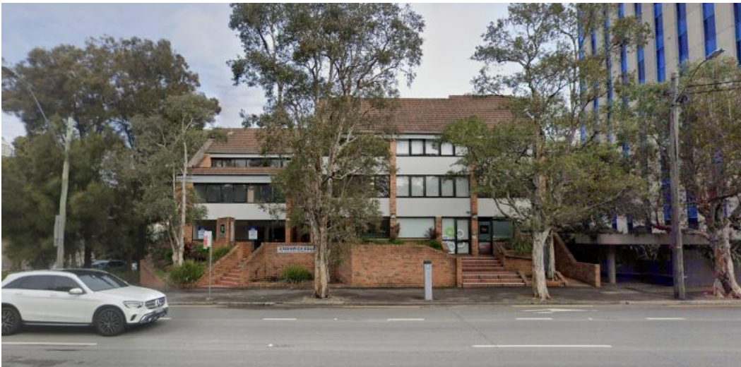
Figure 3: Existing building at 130-134 Pacific Highway (Source: Google Maps)
