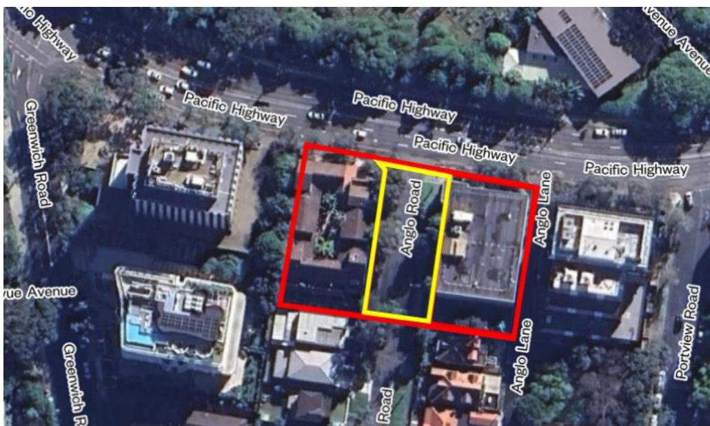
Figure 1: Aerial image of the site – subject site shown red and 'Anglo Road land' shown yellow ( Source: Mecone Mosaic )
